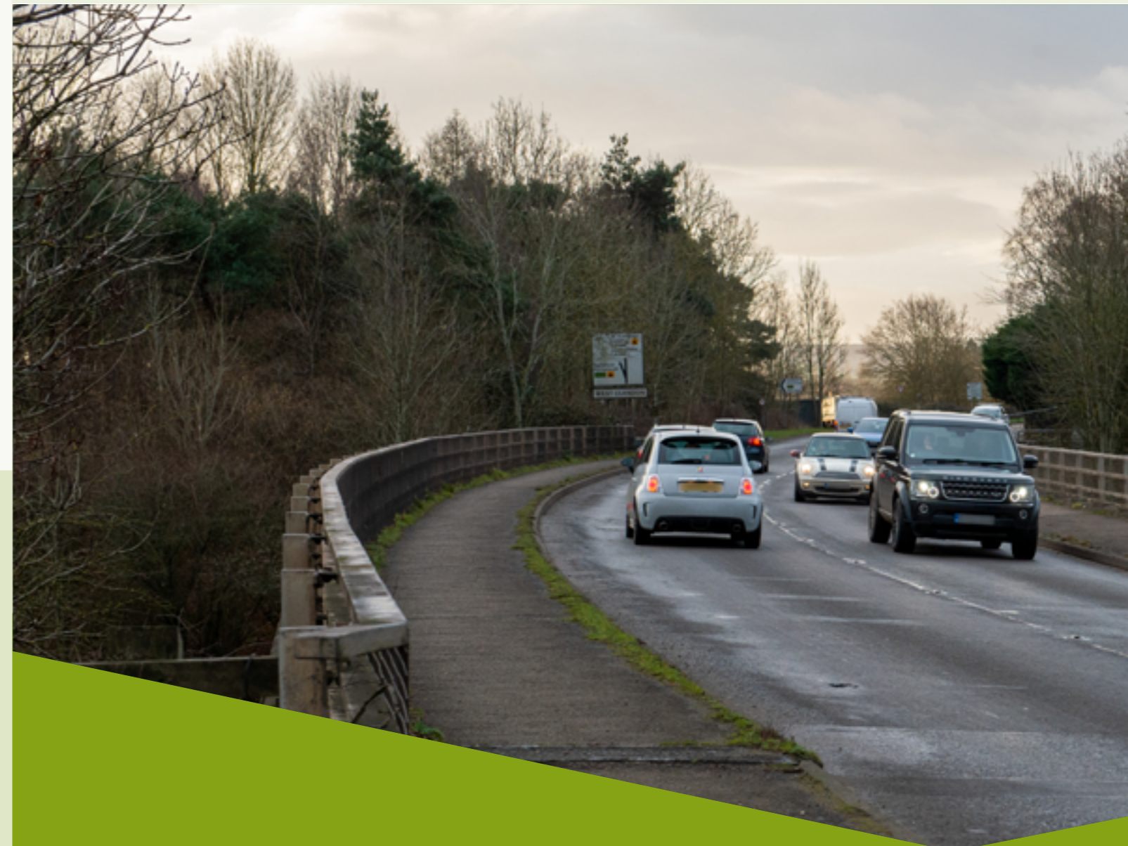
Picture: The A303
